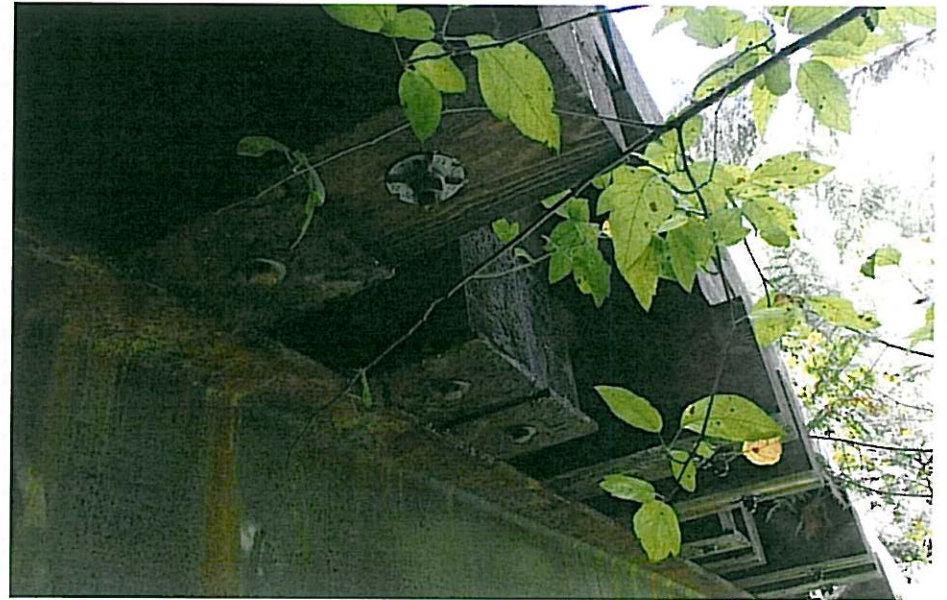
CK-2269 Deck & Girder Bolts
